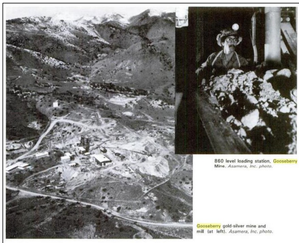
Figure 3: Images of historic production (Schilling, NBMG 1984).
