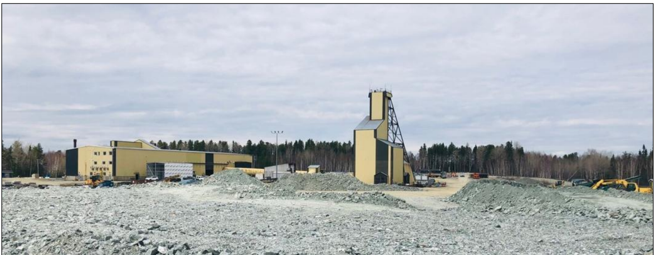
Photo 18.2-1 As-built Beacon mill and mine shaft (October 2025).
