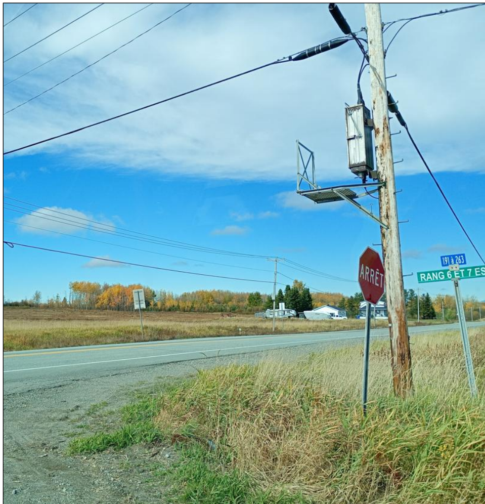
Photo 5.1-1 Swanson Highway 397 access via gravel road (October 2025).
